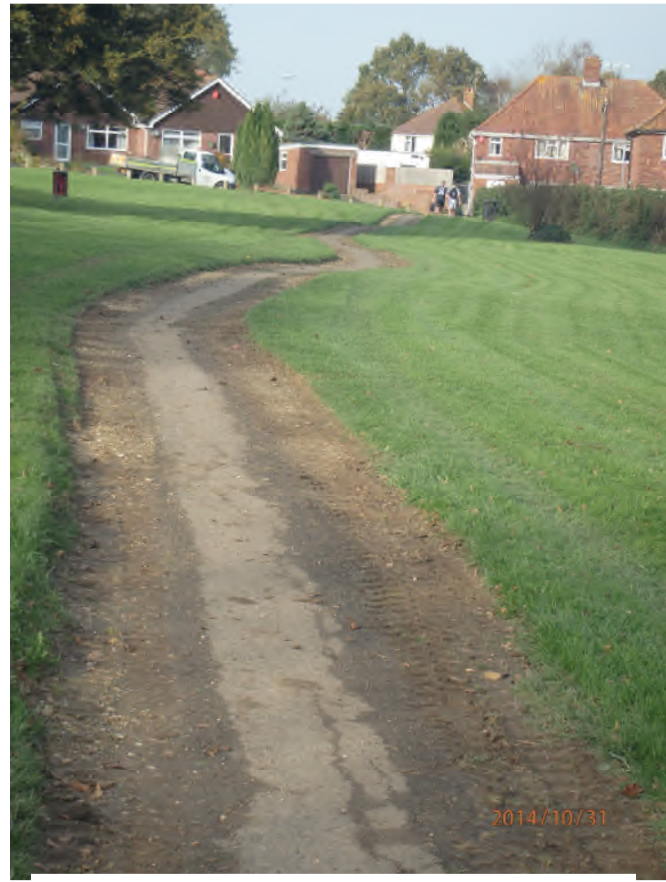
RHS of park, looking towards Allingham Road.
